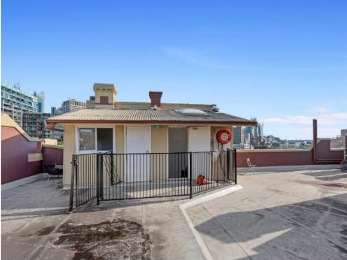
Figure 26: Views from roof terrace of 80 Oxford Street
