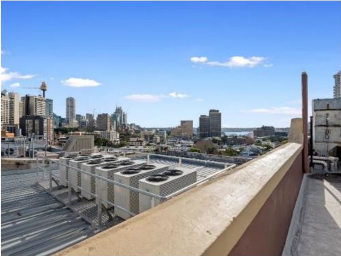
Figure 25: Views from roof terrace of 80 Oxford Street
